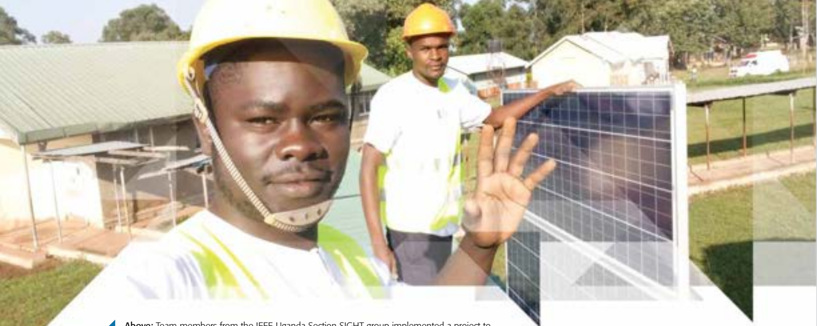
▲ Above: Team members from the IEEE Uganda Section SIGHT group implemented a project to install a solar energy system to facilitate the healthcare services at the Mukujju Health Center IV.
